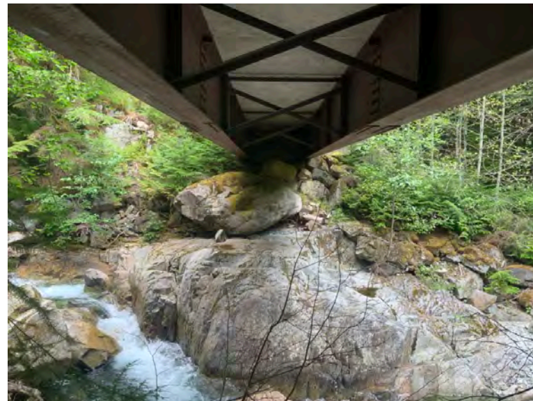
Left Bank Abutment when facing downstream
