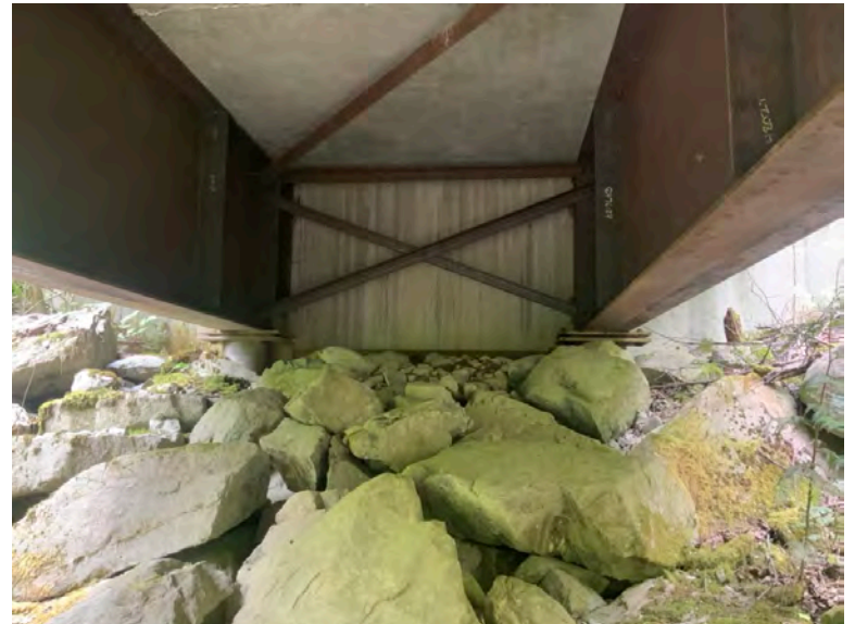
Right Bank Abutment when facing downstream
