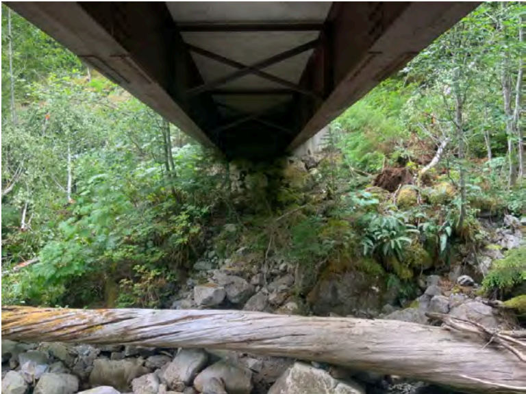
Right Bank Abutment when facing downstream
